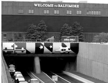
The Fort McHenry Tunnel in Baltimore, Maryland. MARYLAND TRANSPORTATION AUTHORITY
