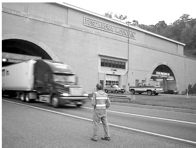
Figure 2. East end of Tuscarora Mountain Tunnel.
