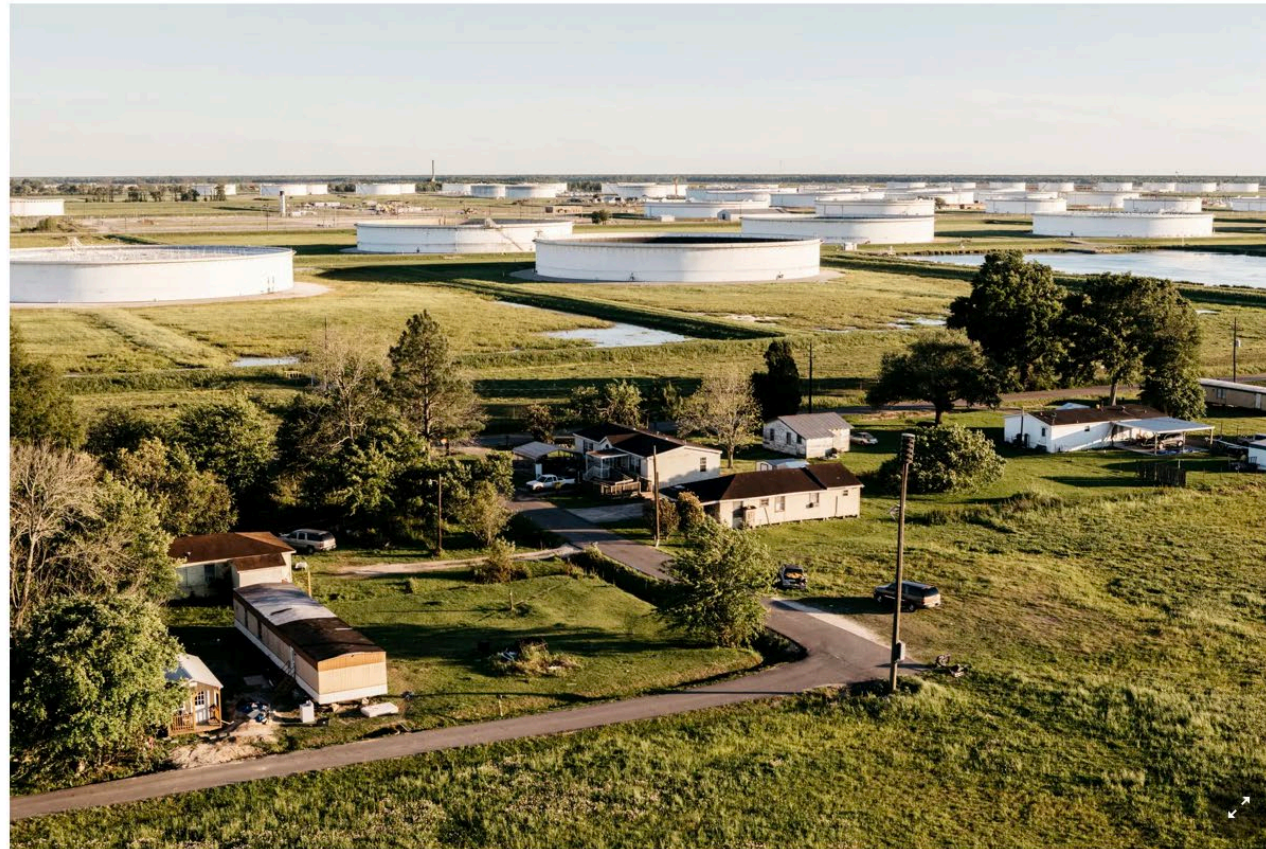
St. James, La., one of several Mississippi River towns dotted by chemical plants and oil refineries. William Widmer for The New York Times
